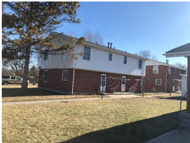
Photograph 9: View of rear entrance to buildings fronting Third Street.
