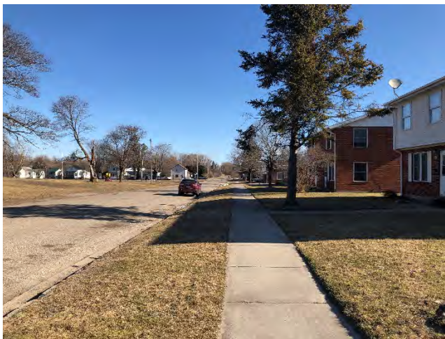
Photograph 2: Near the southwest corner looking north along North F Street.
